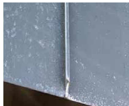
Examples of salt deposits on façades, seams and drip edges
